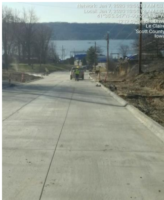
Blowing out the saw joints for Tar
