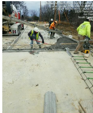
Pouring North end of Phase III
