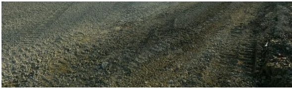
Placing rock to make driveways accessible again.
