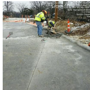
Pouring Phase III East Basins
